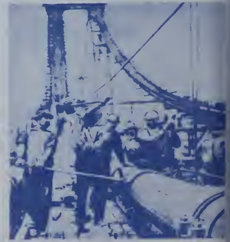
The 19 strands in each cable make a bundle 15¼ inches thick. After being strung, the strands were compressed into cylindrical form by large clamp tongs.
